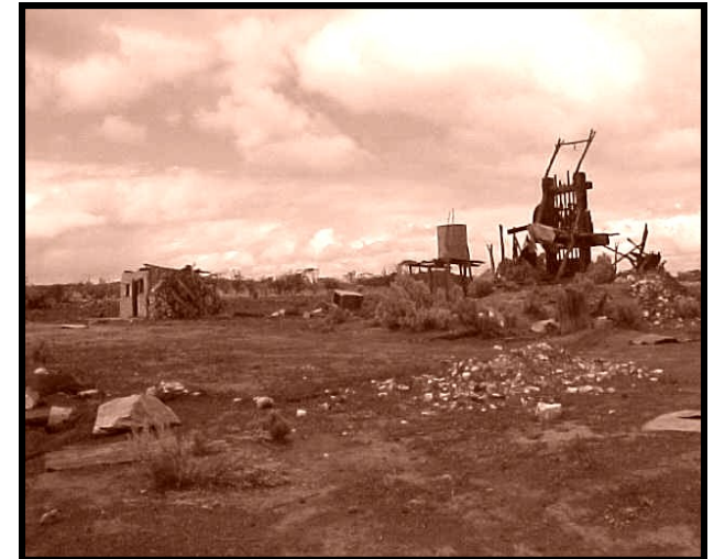
Golden Valley Battery site
